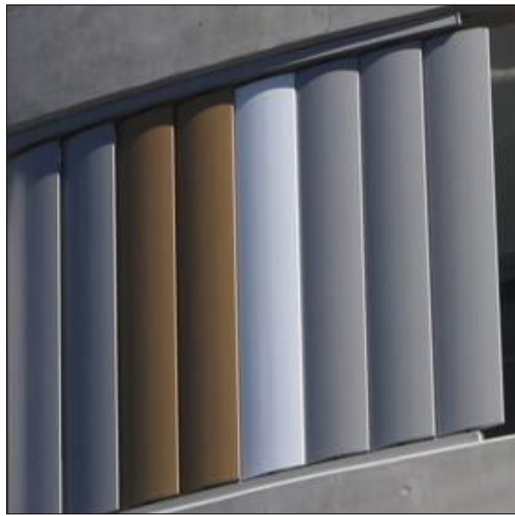
05 - Aluminium Louvre Fins powdercoat to match Dulux Pale Oriental or similar
